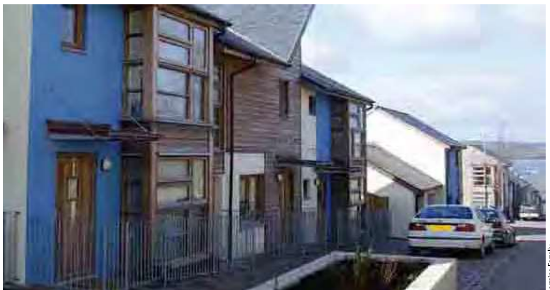
Figure 2.3 A residential environment showing distinctive character.
