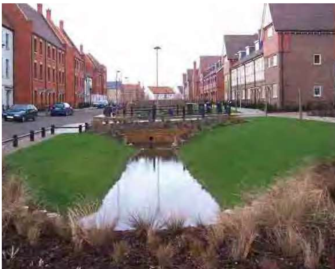
Figure 11.5 Sustainable drainage systems can form an integral and attractive part of the street.
